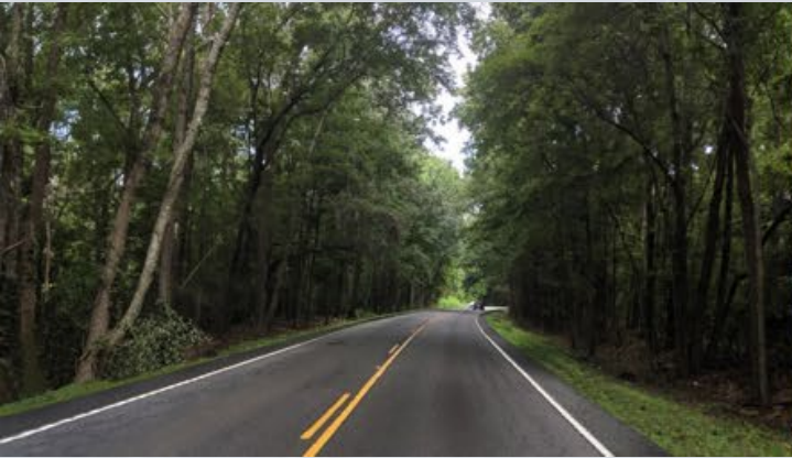
Rural Road Safety
